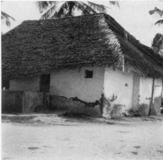
b. — Village mosque, Msasani, near Dar es Salaam.
